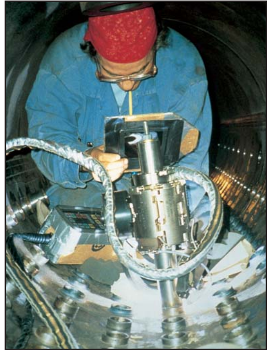
Model 81 in AVC/tilt version welding inside mud drum
