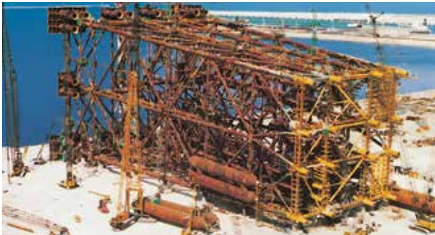
Offshore plant construction: platform
