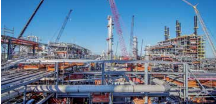
Mechanical contracting and process plant engineering
